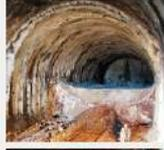
Mechanical or hand excavation in poor quality rock masses (no blasting) results in minimal disturbance to the surrounding rock mass.
