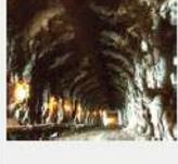
Where squeezing problems result in significant floor heave, disturbance can be severe unless a temporary invert, as shown in the photograph, is placed.
