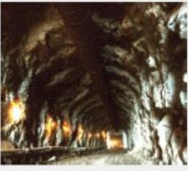
Excellent quality controlled blasting or excavation by Tunnel Boring Machine results in minimal disturbance to the confined rock mass surrounding a tunnel.
